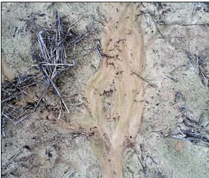
Fig 42. Evidence of water running across top of sand rather than soaking in, May 11, 2016
